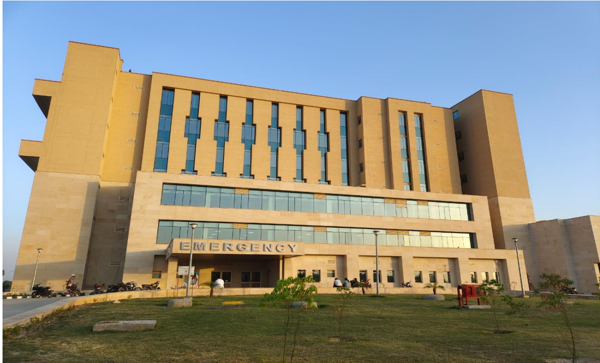
IPD Building (Block A) Emergency Services
