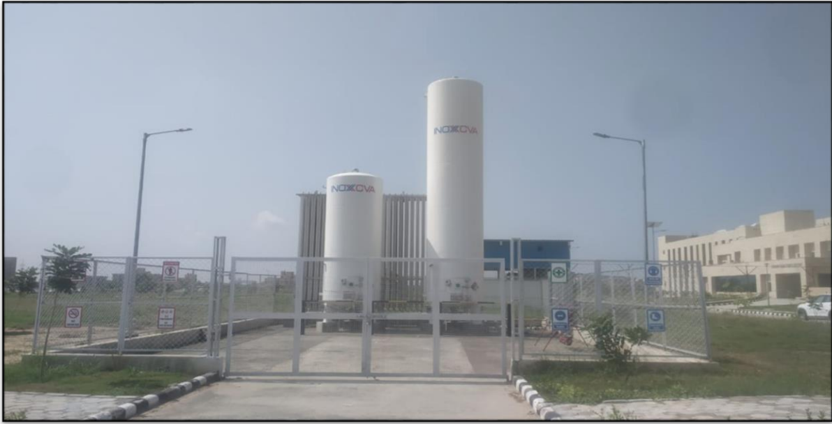
Liquid Medical Oxygen Tanks of 20 KL + 10k KL capacity for continuous supply of Oxygen to ICU, MICU, NICU, Emergency, Wards
